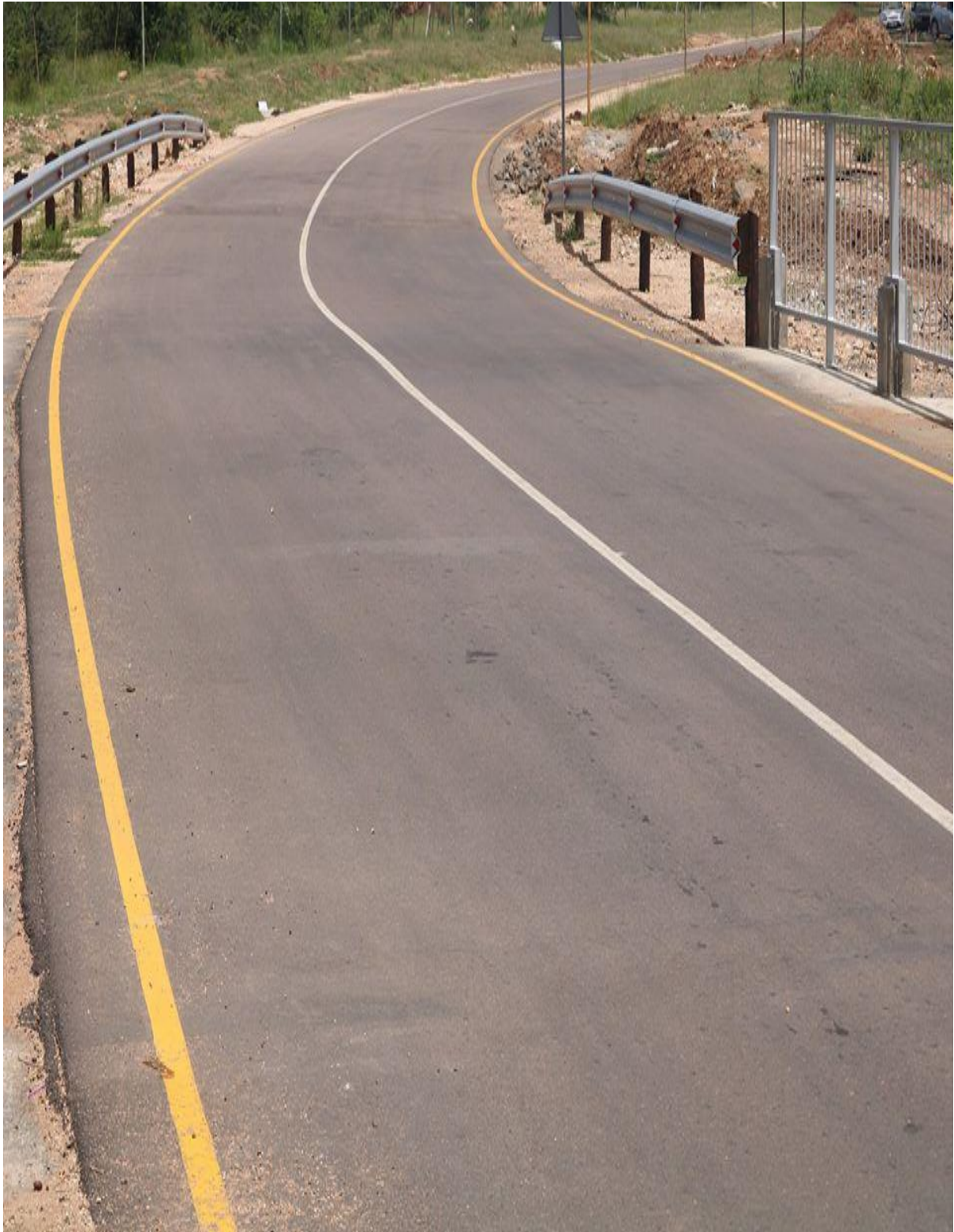
Tshelang Gape to R71 road upgrade project
